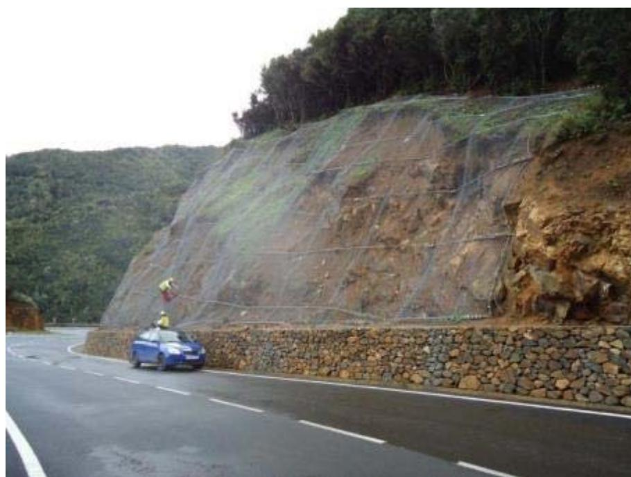
*Picture 28:Implementation of a stabilizing mesh*
