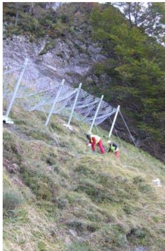
*Picture 32:Installation of the anti-slide barriers*
