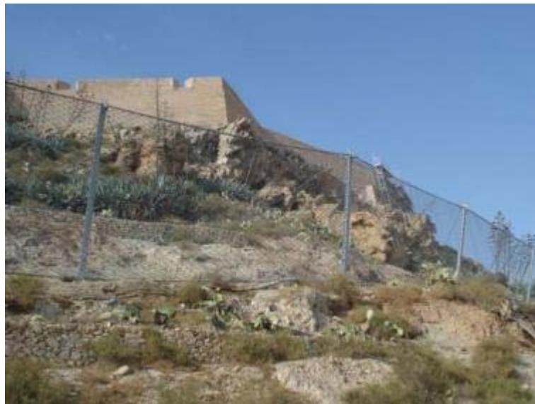
*Picture 3: Situation after the installation of dynamic anti-landslide barriers*
