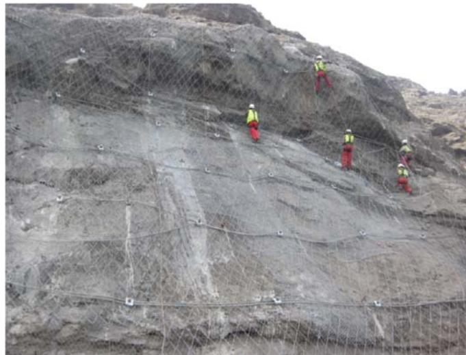
*Picture 21:Implementation of the stabilization mesh*
