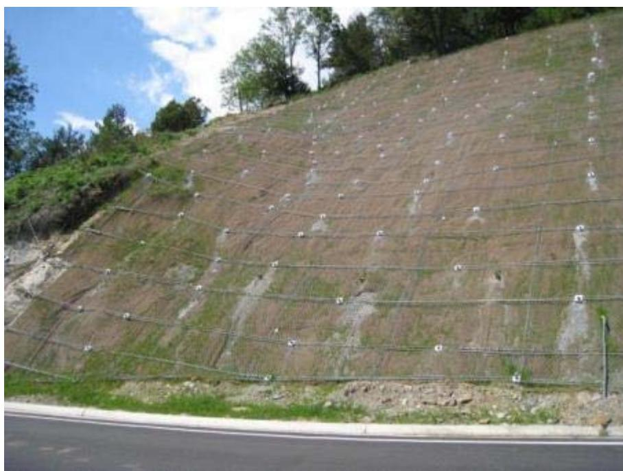
*Picture 36: Installed stabilization mesh*
