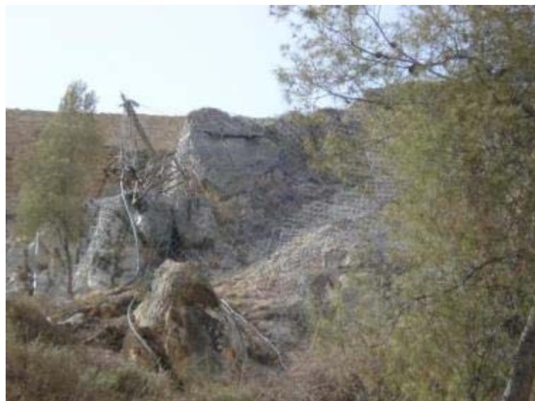
*Picture 8: Progress of the installation of the stabilization mesh*
